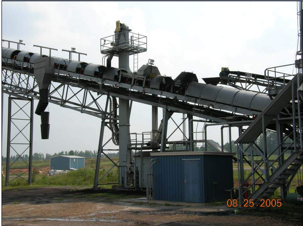
Figure 7. Redundant lines after the EuroSilos
