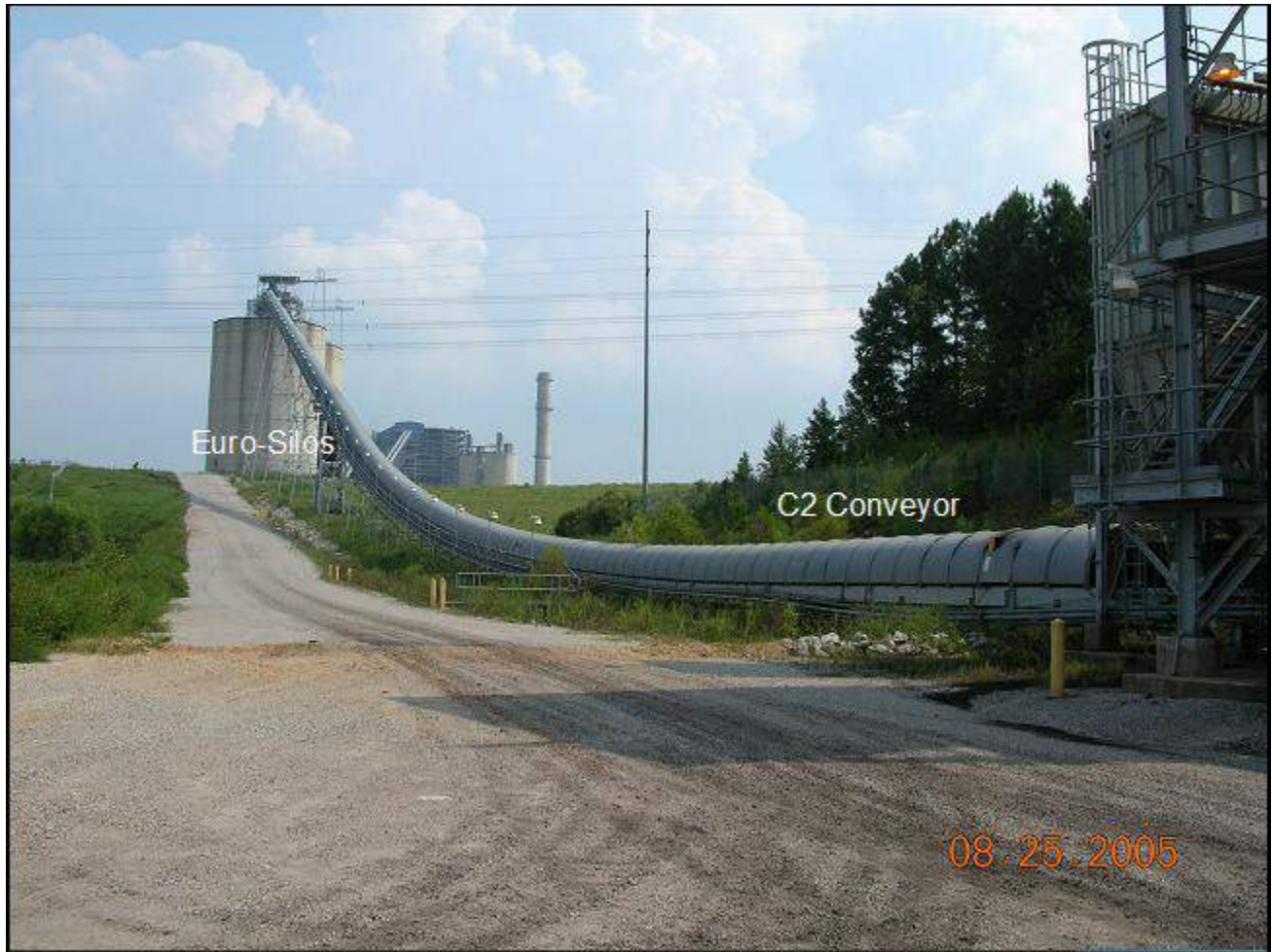
Figure 5. Coal transfer points before the generation plant
