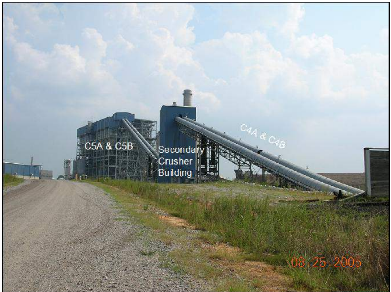
Figure 6. Redundant lines after the EuroSilos
