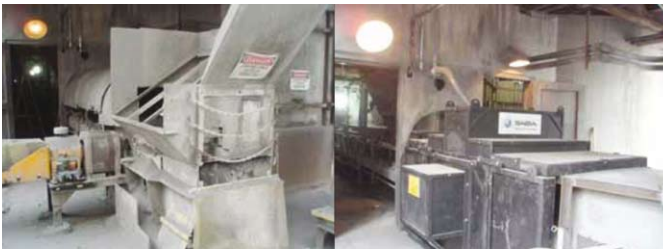
Figure 2. Lafarge Whitehall analyser location before and after installation.
