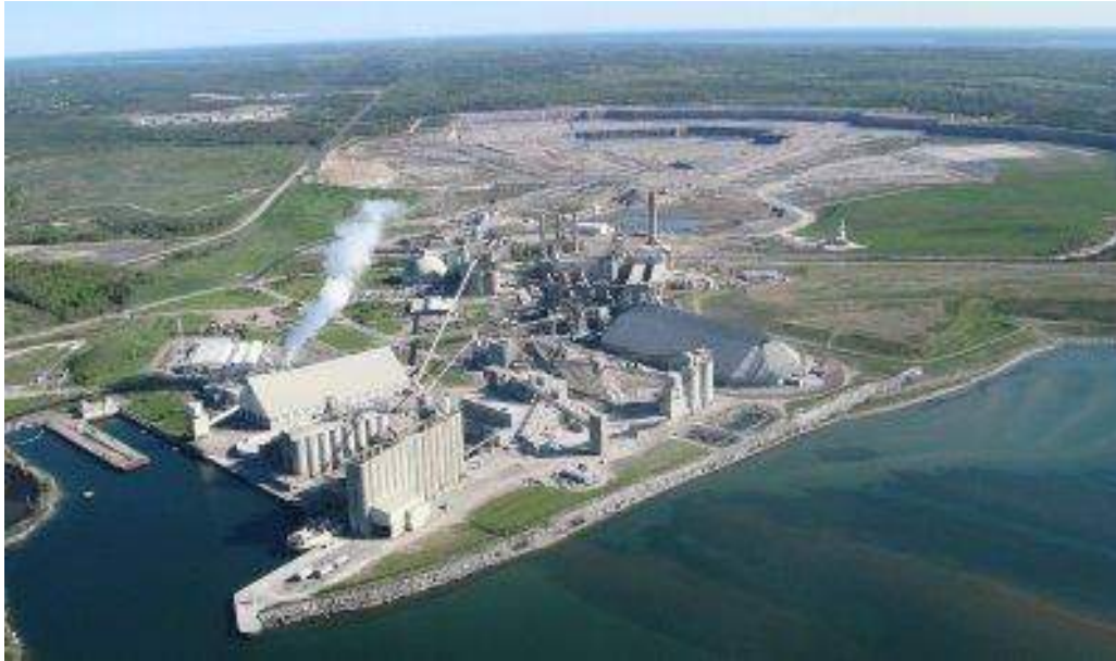
Figure 5. Alpena Cement Plant
